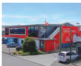
Fujitsu General New Zealand Ltd. (Nowa Zelandia)
